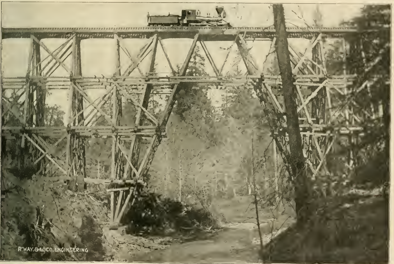
SCENE ON EUREKA & KLAMATH RIVER RAILROAD, CALIFORNIA. (Bridge 500 feet long, 110 feet high, contains 500,000 feet of timber.)
